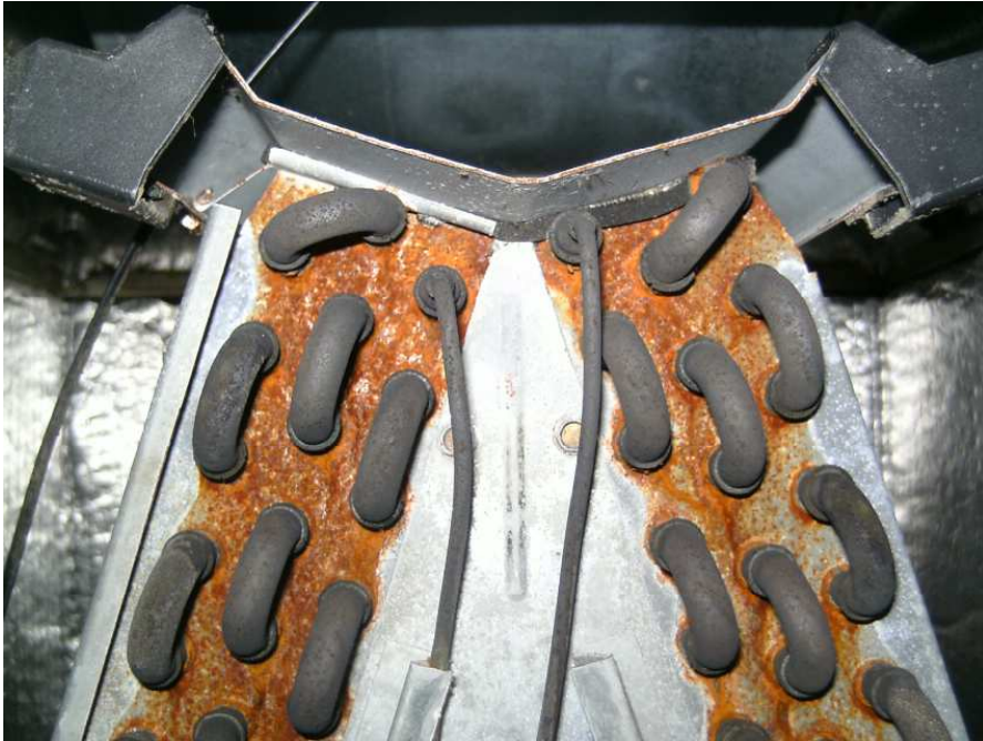
Blackened Cooper Coil in Air Handler
