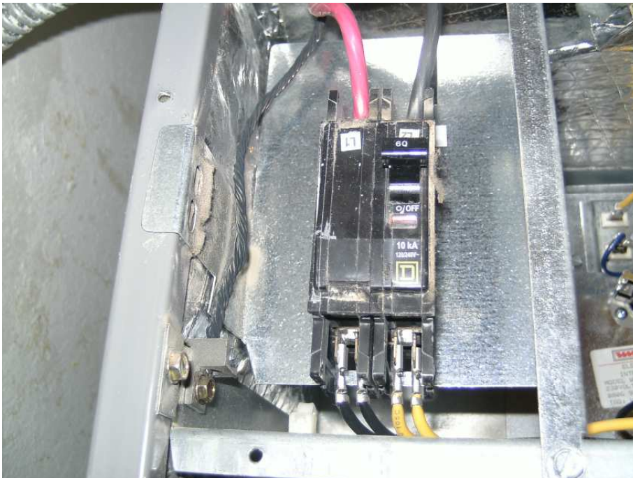
Air Conditioning Air Handler – Blackened Copper Wiring
